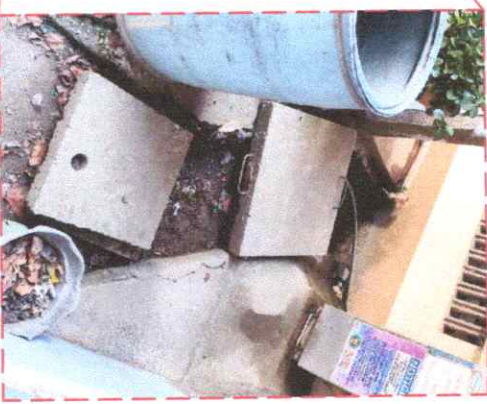
DRAINAGE OPENING IS OBSTRUCTED BY A BROKEN CONCRETE SLAB AND DEBRIS CAUSES SURFACE WATER ACCUMULATION AND FLOODING DURING HEAVY RAIN
