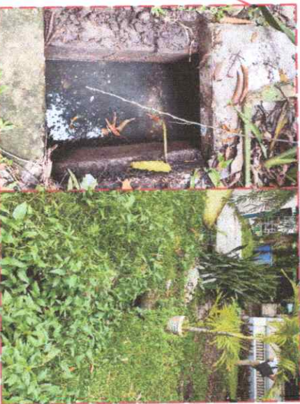
DRAINAGE OUTLET OPENING TO GROUND
